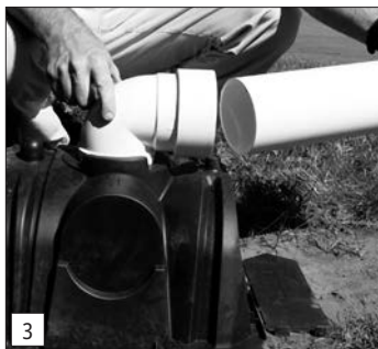
Connect inlet pipe.
