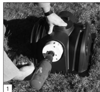
Drill endcap on side or top.
