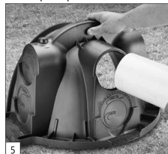
Install splash plate.
