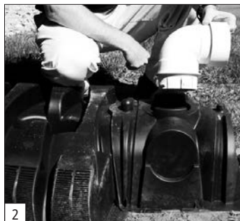
Insert Quick4 Plus Periscope.
