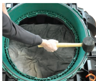
Use mallet to engage the rest of the tabs.
