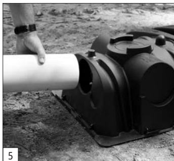
Insert inlet pipe.
